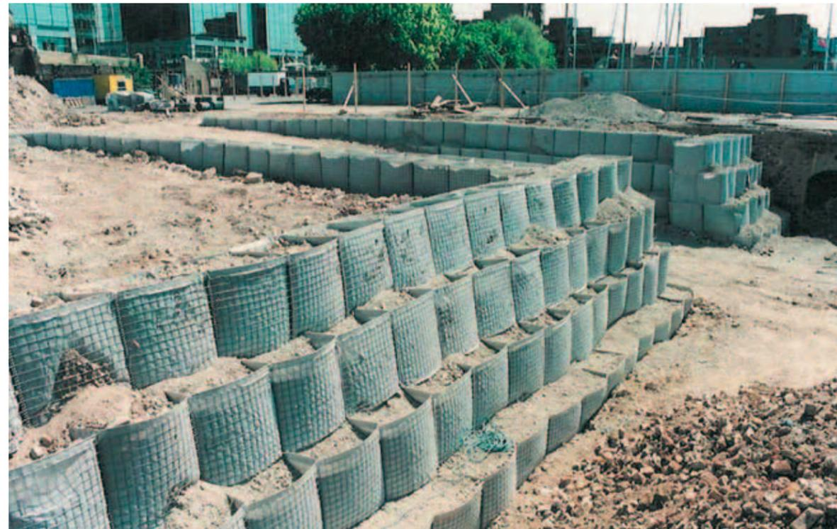
Betafence Weldmesh® Bastions are factory lined internally with a non woven geotextile membrane to the perimeter mesh panels of the unit, allowing for the use of suitable selected granular fills to ensure compaction of the materials without any settlement.
