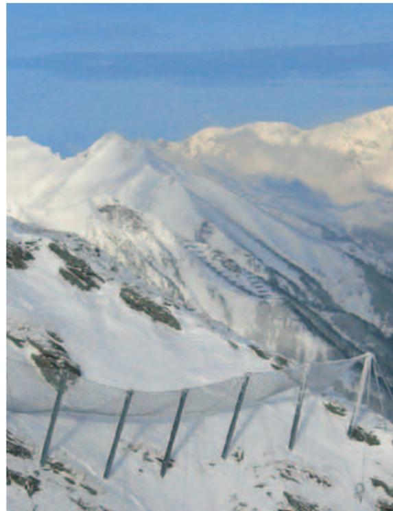
The avalanche protection systems by Trumer Schutzbauten utilize the flexible nature and high strength of the Omega-Net to prevent avalanches in their first stage of occurrence. This means the hazard is essentially removed prior to the start of an avalanche and not just mitigated once it has occurred.
