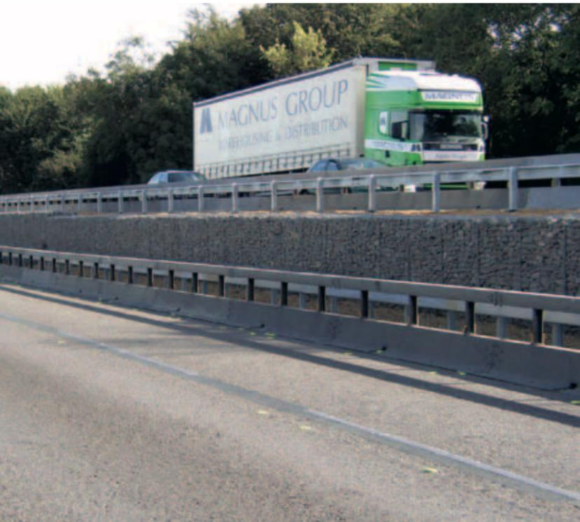
Betafence Weldmesh® Gabions are wire mesh baskets formed by connecting individual panels of mesh with helical spirals on the vertical edge wires creating an open series of box compartments that fold in a concertina fashion to be flat packed. Lids and bases are sometimes supplied loose with helical spiral binders to connect the top and bottom of the open cells along one edge. Alternatively they may be factory fitted where practical for ease of transportation.
