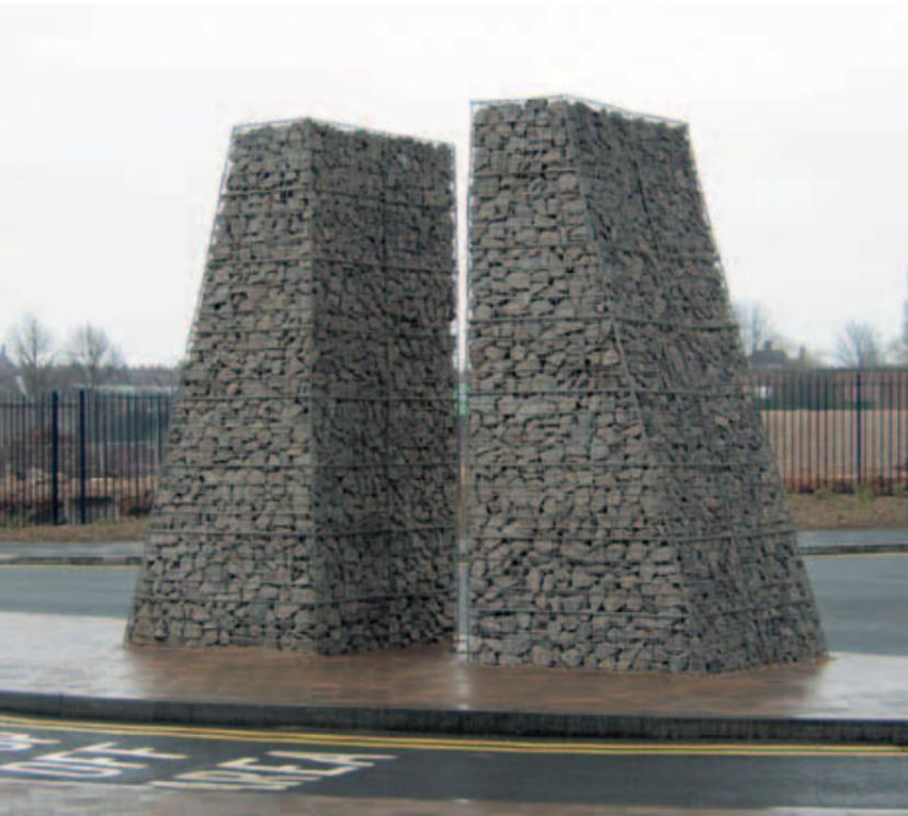
Betafence Weldmesh® Trapions are a form of Gabion manufactured from welded wire mesh panels with either one or both faces inclined at varying angles to the horizontal dependant upon the unit's height. They are supplied in lengths of 1, 2 or 3m or part lengths thereof, and pre-assembled with helical spirals for flat packing and ease of transportation to site.
